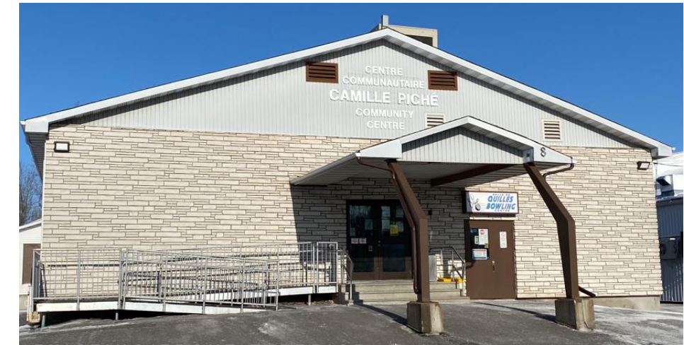
EXISTING FRONT EXTERIOR
